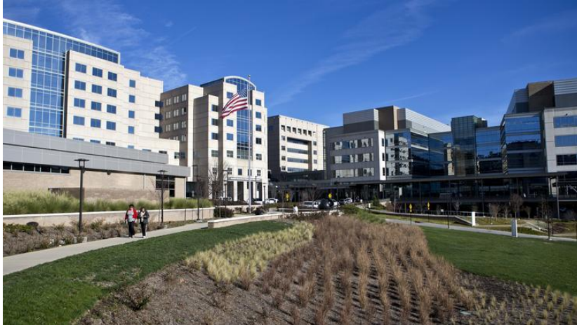
UNC Medical Center in Chapel Hill
